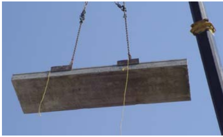
(Above) Pre-cast hollow-core plank (Right) Interior Bearing Wall Detail provided by Nitterhouse Concrete
