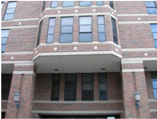
(Above) Reinforced masonry wall
